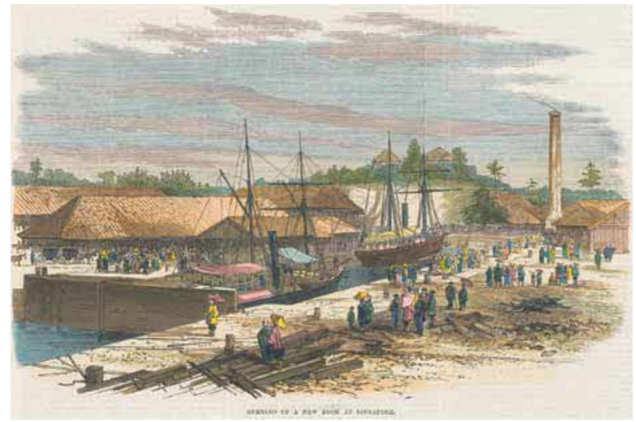
This wood-engraved print shows the opening of Victoria Dock at New Harbour by then Governor Harry St. George Ord on 17 October 1868. Courtesy of National Museum of Singapore, National Heritage Board.
